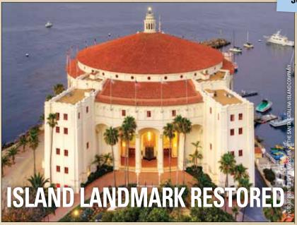
■ AVALON, CALIFORNIA — L.A.-based Spectra Company's facade restoration of Catalina Casino, a 12-story Santa Catalina landmark, was a comprehensive preservation project including lead-based paint remediation, epoxy injection, spall/crack repair, ornamental stone repair/replication, door/window restoration and a complete waterproofing with sealants and caulking.
