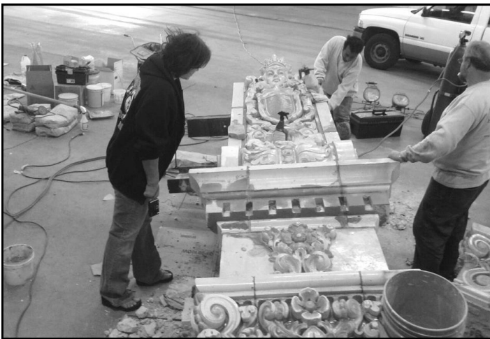
In process—cleanup, filling in and painting the terra cotta details
